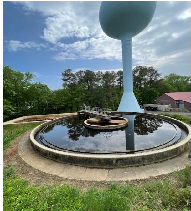
In fact, iron is problematic in our aquifers and the first thing our water treatment facility does when water is pumped to the facility is remove iron. The plant uses a device called a clarifier that separates the iron from the water, allowing it to fall into a sump where it is pumped to a retention pond. In an average year, 90,000 gallons of iron sludge is pumped from this retention pond. The device that separates iron from our water is a critical piece of infrastructure.
